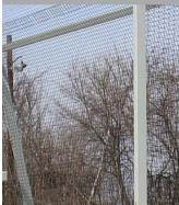
Wind Screen is Welded Wire galvanized and vinyl coated, built to take the harsh environment at landfills.
